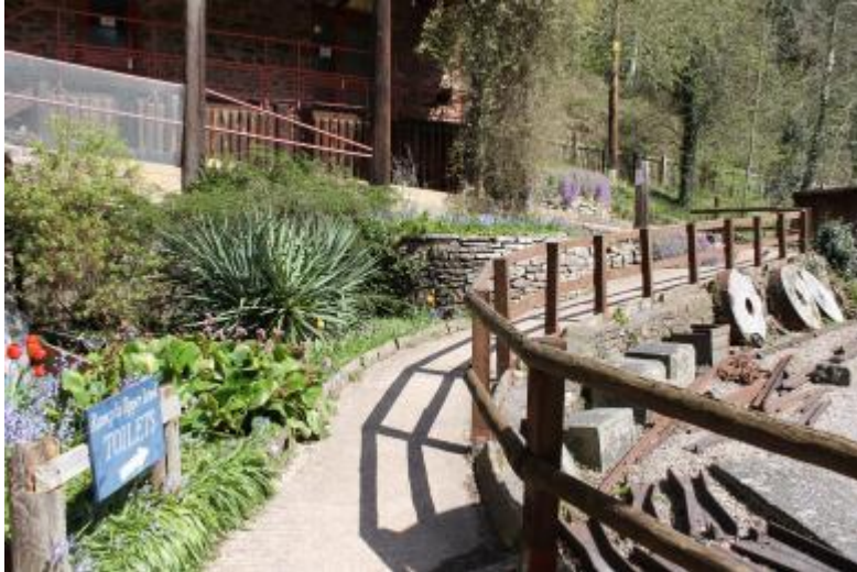
Ramp to 1st floor at rear of building
