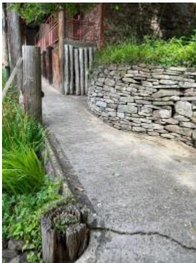
view of ramp going towards toilet block
