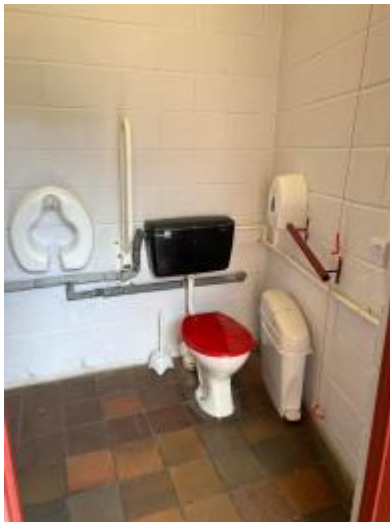
view of disabled toilet
