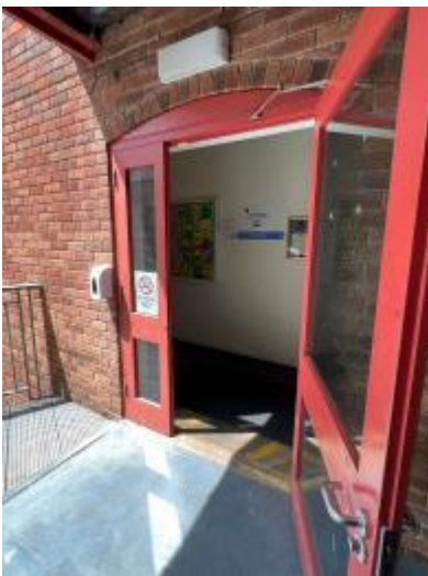
door to corridor for rear entrance to coffee shop
